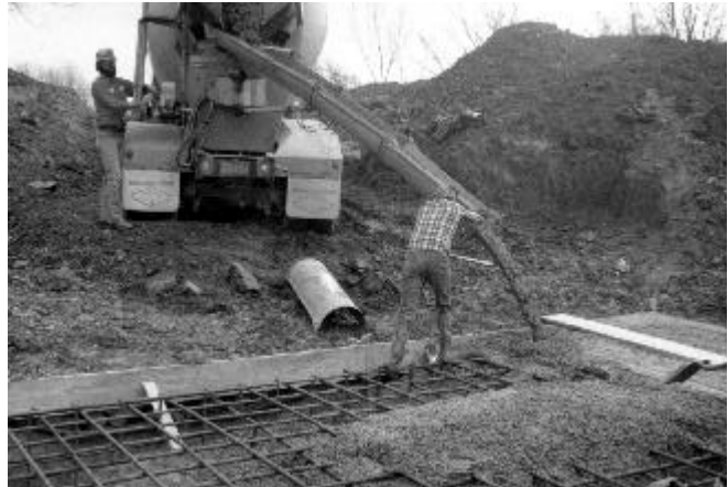
Workers forming concrete cap. Photo provided by Oklahoma Conservation Commission.
